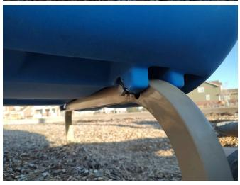
The tube slide on the west side of the composite structure has a number of bolts that seem loose due to the connection inserts being stripped out. Recommend continued inspection and possible replacement of slide exit if gaps develop between sections (CPSC 2.5.2)(Priority 3 Hazard)
