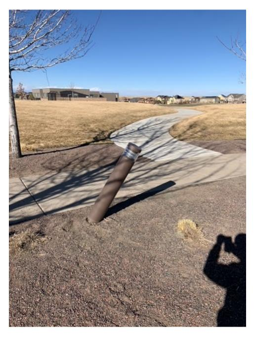
After speaking with Full Spectrum, their technician believes the damage was likely caused by a snowplow, although it's challenging to determine conclusively. They mentioned that the force required to cause such damage could be from either kicking it over or from a plow of some sort.
